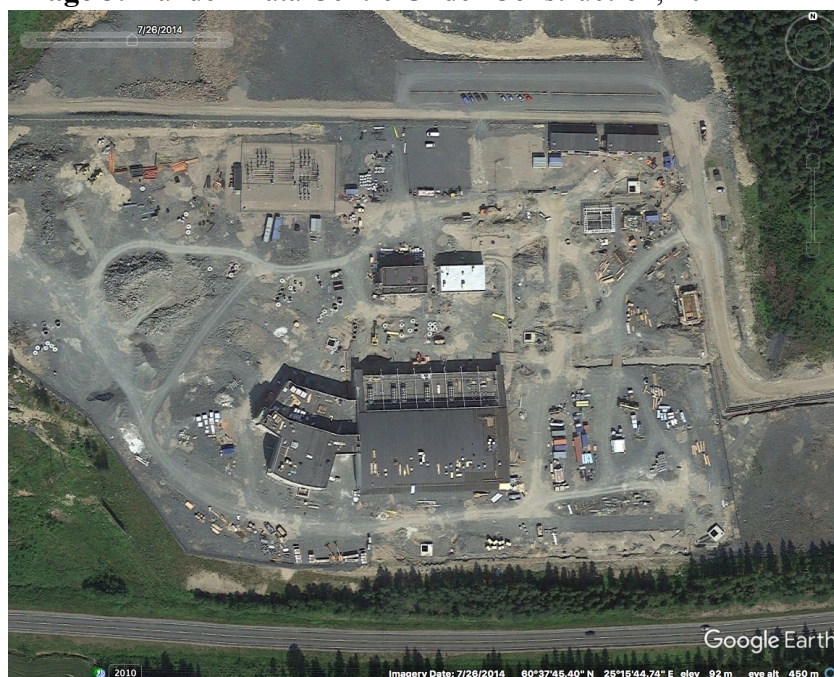
Image 3. Yandex Data Centre Under Construction, 2014
