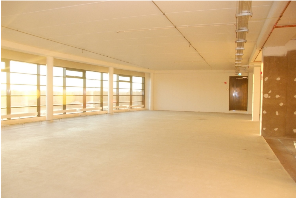
Image 9. One of the four empty floors in the main administrative building of the Yandex data centre.
